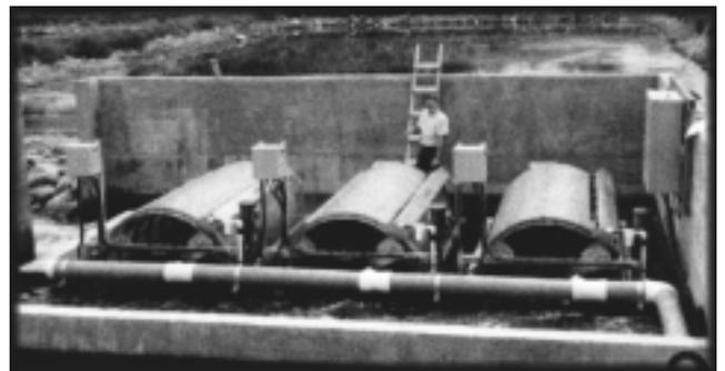
3 models 1607-24 with flow capacity = 16000 gpm
